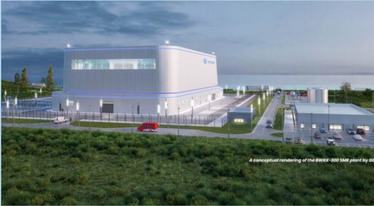
Darlington 300MW SMR Generating Station, Ontario
